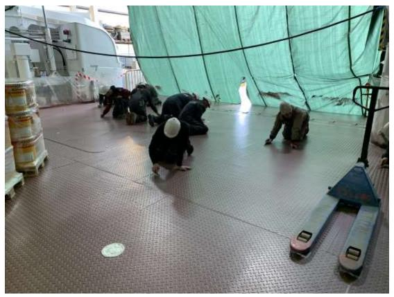
Cleaning /removal of minor locations with steel particles "abrasives from blast cleaning".
